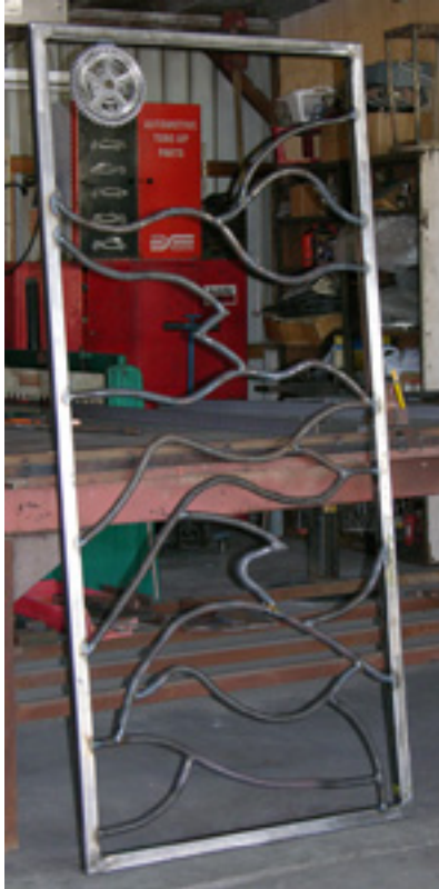
Cruisin's door frame is nearly completed
